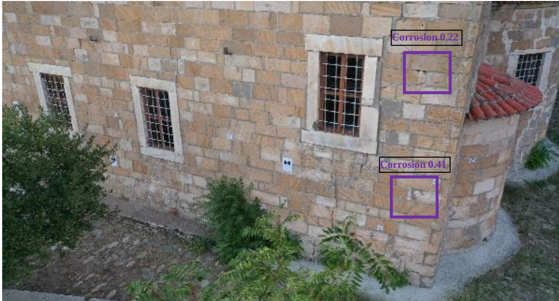
Figure 3: Conceptual results from UAV Mission 1 – Asset (church in Mytilene) with defect detection using multiclass object detection model and annotations highlighting corrosion.
