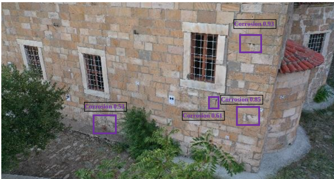
Figure 4: Conceptual results from UAV Mission 2 – Asset (church in Mytilene) with defect detection using multiclass object detection model and annotations highlighting corrosion areas. The increased number and extent of these areas in comparison with the results of UAV Mission 1, suggest a potential worsening of the asset's condition.
