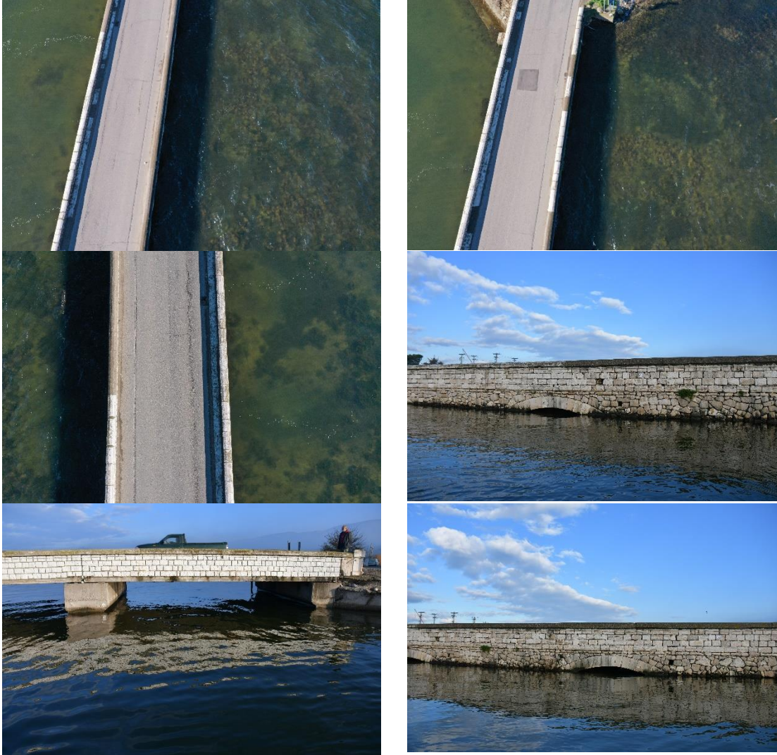
Figure 2: Photos of the stone bridge in Aitoliko
