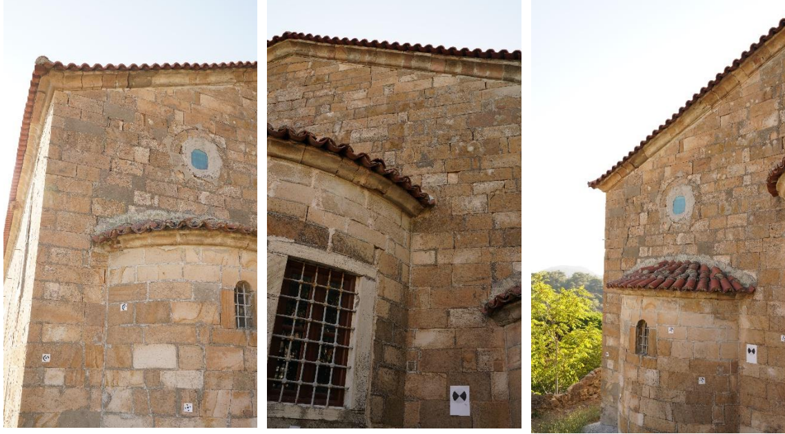
Figure 4: Photos from an old building in Mytilene
